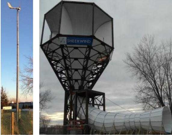
Figure 5 Fielded INVELOX demo (right) and Conventional turbine-tower system (left) under evaluation in Chaska, Minnesota
